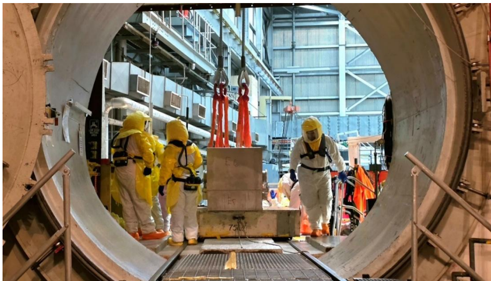
Fuel assembly is moved through the equipment hatch using Holtec's Fuel Transfer Canister for storage in the spent fuel pool.
