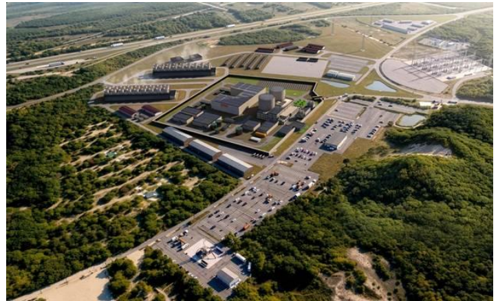
The Pioneer 1 & 2 units will add 680 MWe to the 805 MWe output to the Palisades plant
