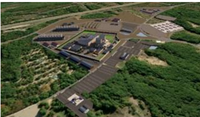
Pioneer 1 & 2 rendering overlaid on the recently cleared land at the Palisades Nuclear Plant in Covert, Michigan
