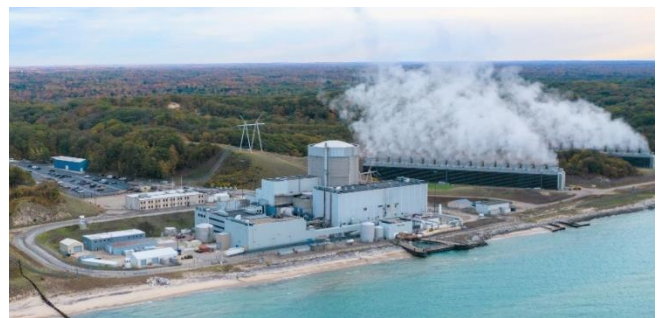
Palisades Nuclear Plant, Covert, Michigan
