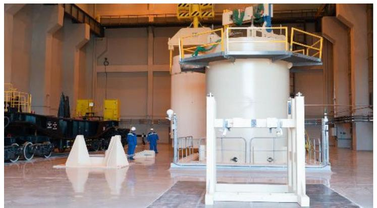
*Central Storage Facility: HI-STAR and the Canister Transfer Device in the Cask Receiving Building*
