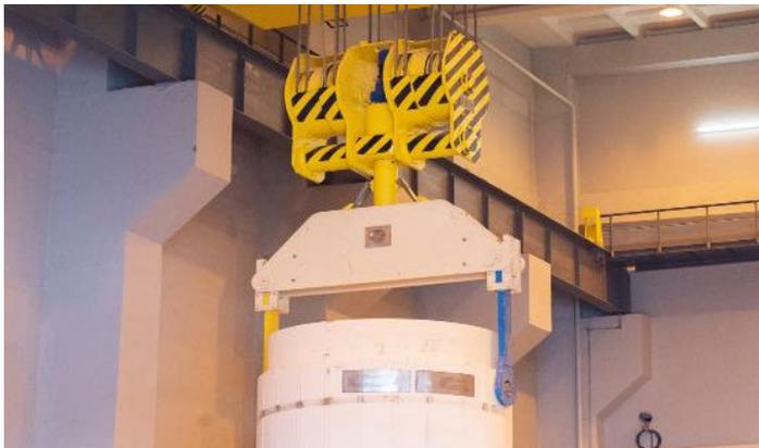
*Central Storage Facility: HI-STAR 190 Lifted by the Cask Receiving Building's Main Crane Using the HI-STAR Lift Yoke*
