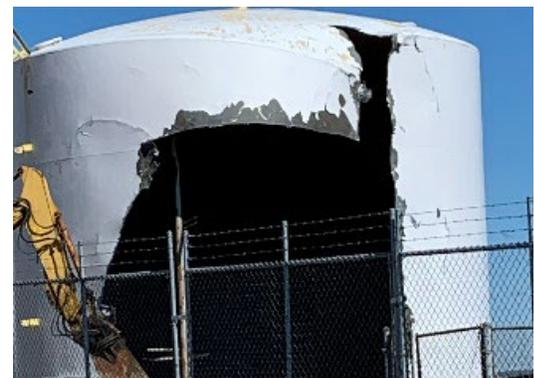
*Firewater Storage Tank, Containing Asbestos in the Paint, is Removed From Pilgrim*
