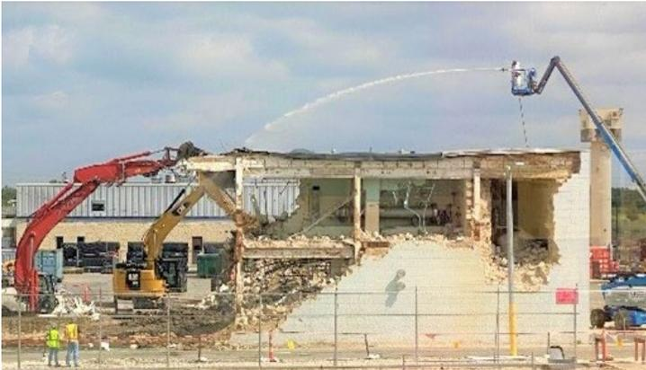
*Demolition of Oyster Creek's Air Ejection Off-Gas Building*
