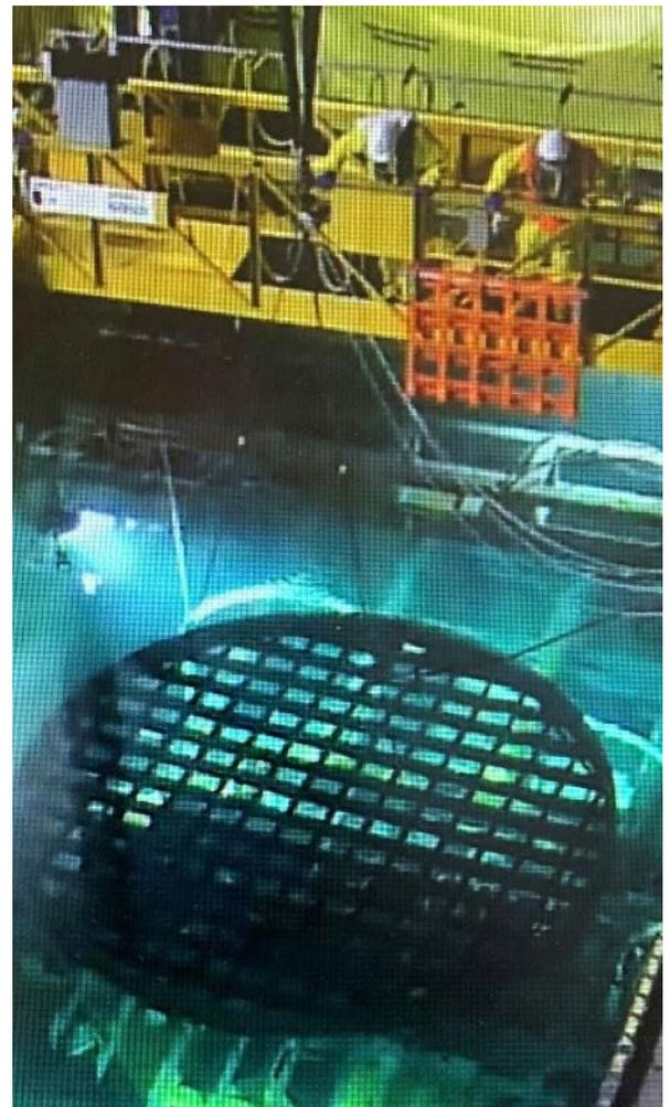
*Top Guide is Prepared for Segmentation as Part of the Reactor Vessel Internals Work at the Pilgrim Decommissioning Site*
