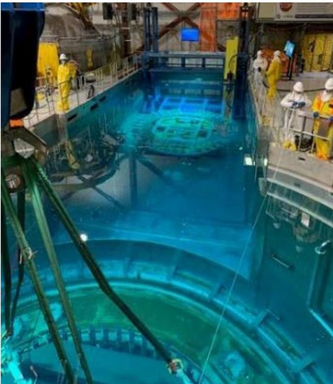
*Segmentation of Reactor Vessel Internals at Pilgrim*
