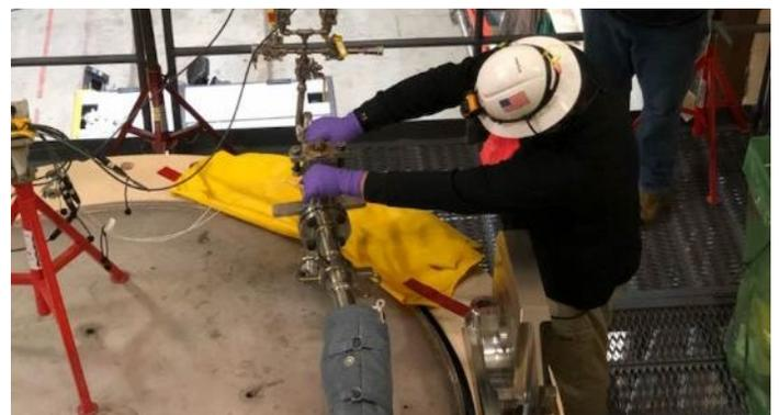
*HI-TRAC Transfer Cask Inner-Shell Being Installed Into the Neutron Shield Cylinder and Bolted Into One Assembly*
