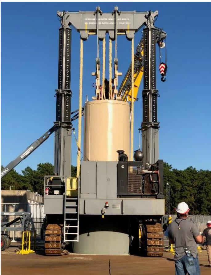
*HI-TRAC Transfer Cask is Placed on Top of the HI-STORM FW Overpack That is Inside the Cask Transfer Pit at Oyster Creek*
