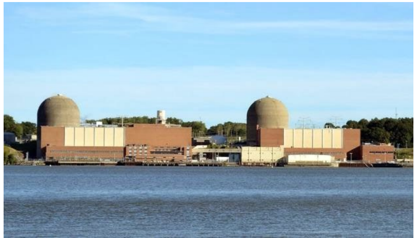
Indian Point Energy Center in Buchanan, New York
