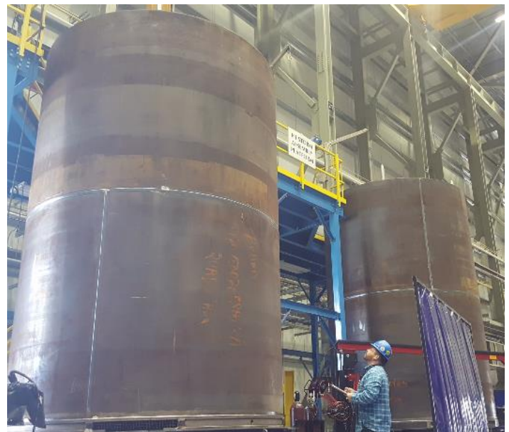
HI-STORM Assembly Platform at Holtec’s Advanced Manufacturing Plant in Camden, NJ
