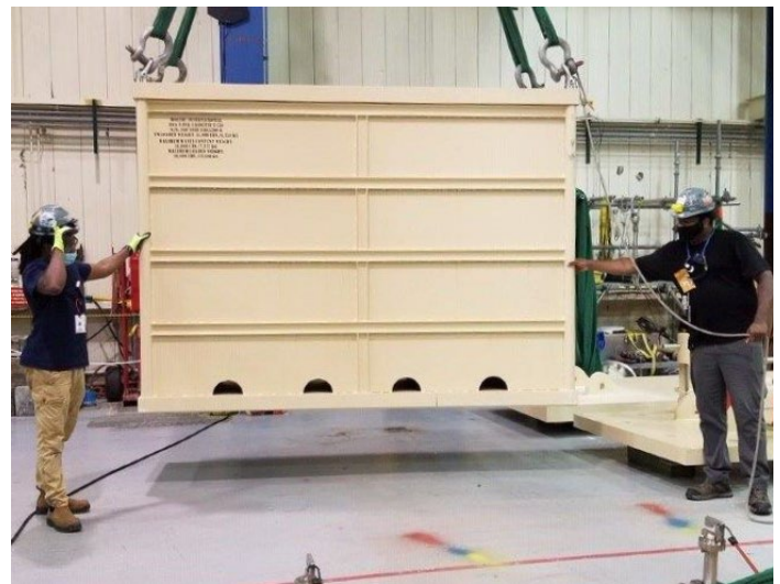
Oyster Creek Associates Safely Move a HI-STAR 330 Class B/C Waste Container to Store Segmented Components
