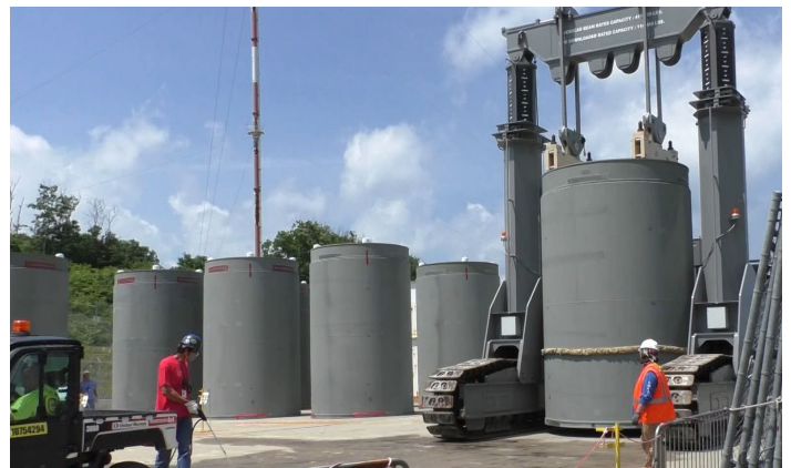
Pilgrim Workers Safely Transport Used Fuel to the ISFSI Pad
