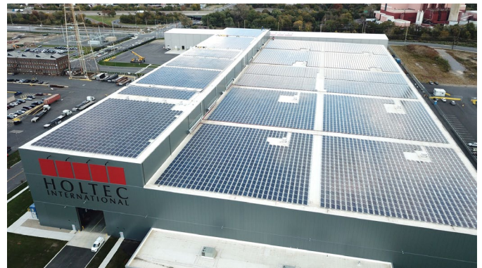
9,000 Solar Modules Provide Electricity to the Advanced Manufacturing Division at the Krishna P. Singh Technology Campus in Camden, NJ
