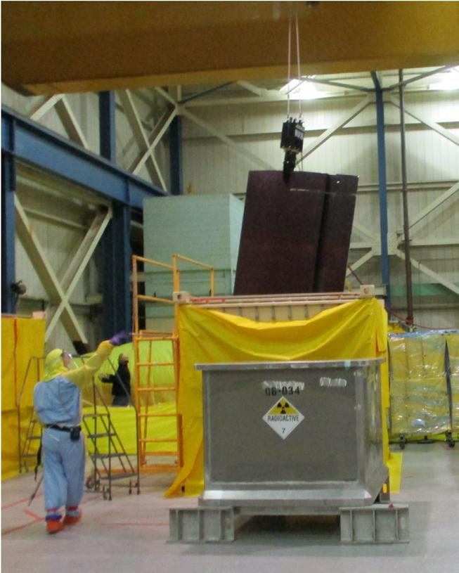
*A Segment of the Steam Dryer Being Loaded into a Waste Storage Container for Disposal Offsite*
