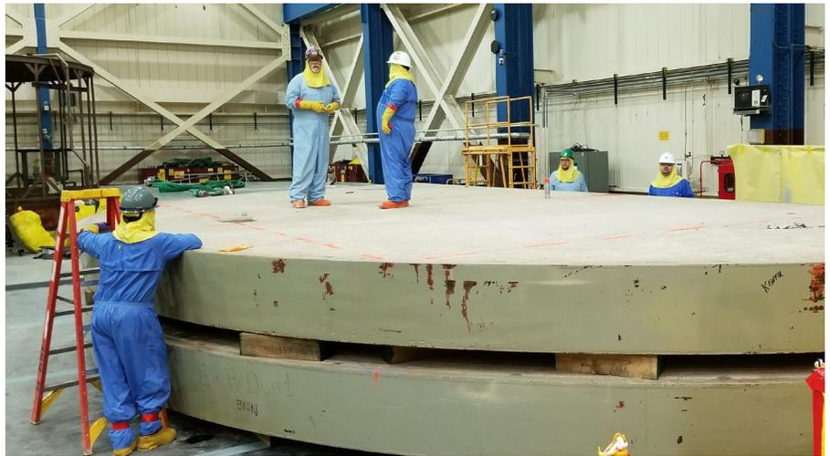
*Oyster Creek Decommissioning Site: Reactor Containment Shield Piece Lowered Through Equipment Hatch (left);
