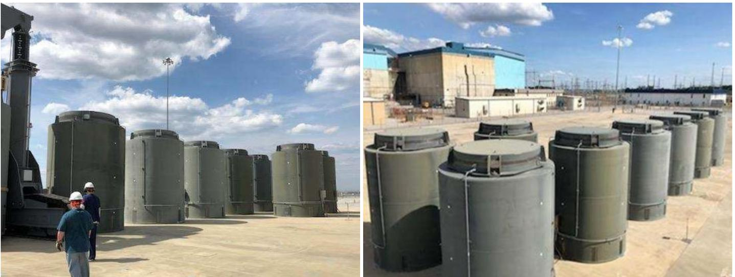
*Holtec's HI-STORM FW Dry Storage Systems Loaded at Dominion Energy's V.C. Summer Nuclear Station*
