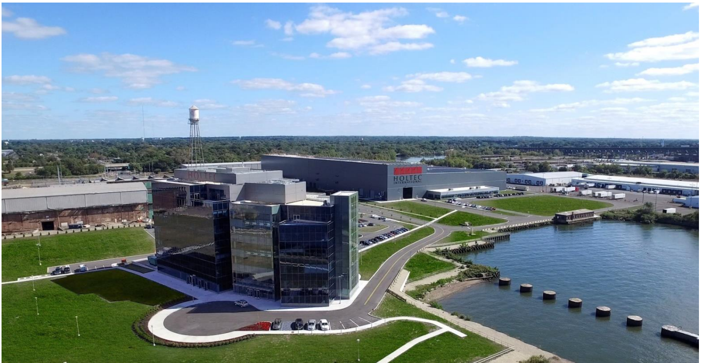
The Campus Located in Camden, New Jersey on the Delaware Riverfront features Holtec's Corporate Engineering Center and two Manufacturing Plants
