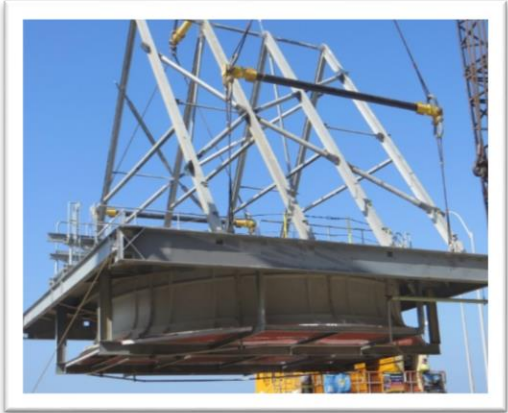
MODULAR CELL BEING HOISTED INTO POSITION.
