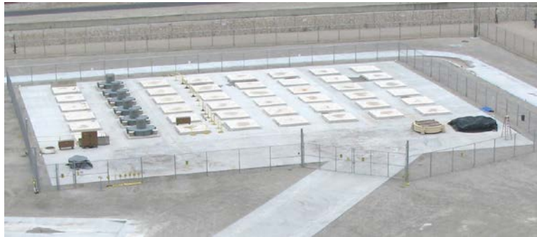
Figure 1: HI-STORM UMAX ISFSI at a US Nuclear Plant
