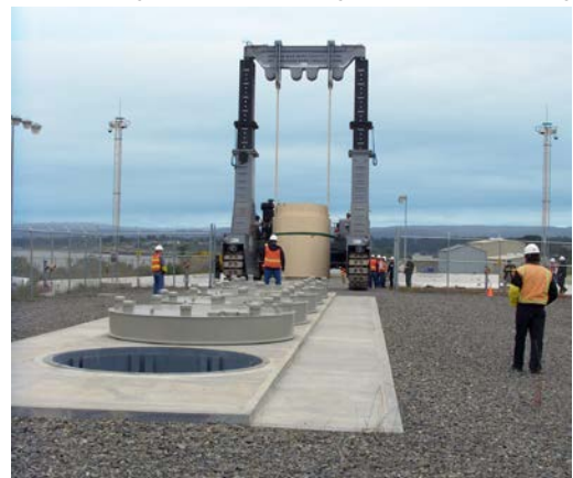
Figure 5: Holtec's Underground Dry Storage System at Humboldt Bay
