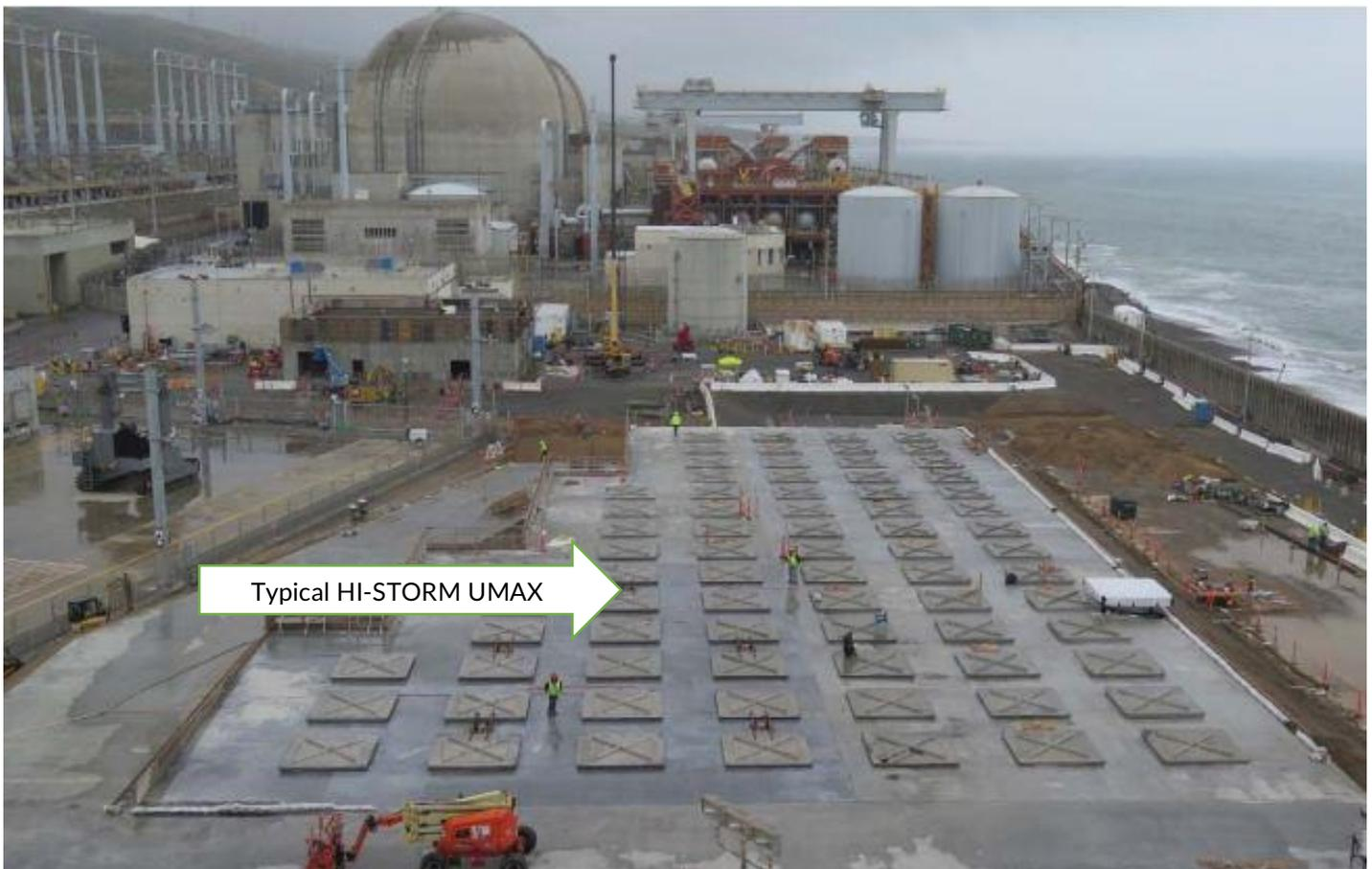
The SONGS ISFSI is unique in that it takes full advantage of the extreme seismic resistance of the in-the-ground HI-STORM UMAX storage modules: The postulated earthquake magnitude, expressed in zero period accelerations, is hair raising 1.5 g in each of the three orthogonal directions.
