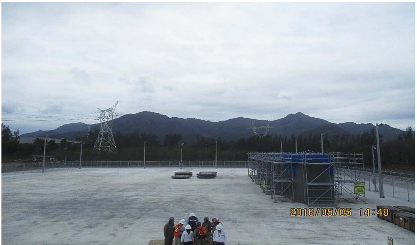
HI-STORM FW Systems on Completed ISFSI Pad at Laguna Verde Nuclear Power Plant
