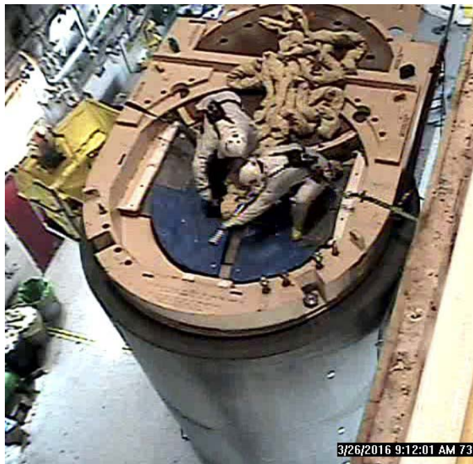
Photo Left: Boilermakers, Casey Pope and Anthony Lambert of TVA, Removing Lifting Cleats from the Loaded HI-STORM FW Dry Storage Cask Photo Right: Installation of threaded plugs into Bolt Holes
