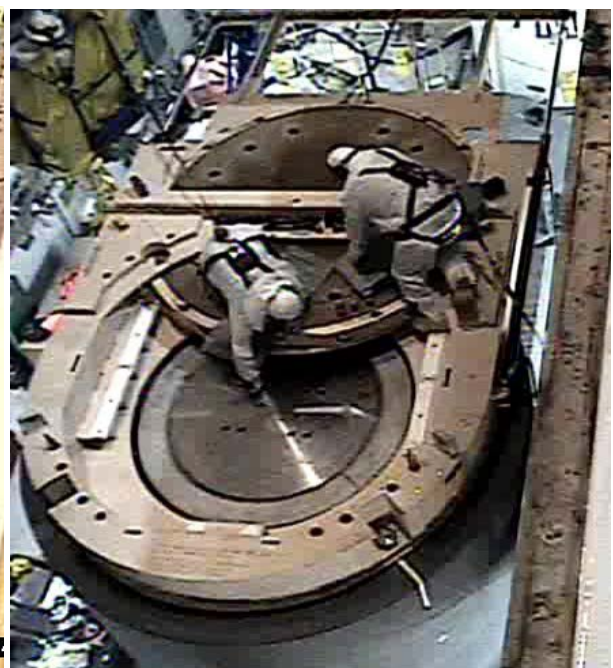
Photo Left: Boilermakers, Casey Pope and Anthony Lambert of TVA, Removing Lifting Cleats from the Loaded HI-STORM FW Dry Storage Cask Photo Right: Installation of threaded plugs into Bolt Holes
