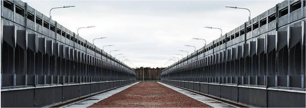
Concrete silos for the storage of more than 42,000 spent fuel bundles built to store fuel safely for over a century.
