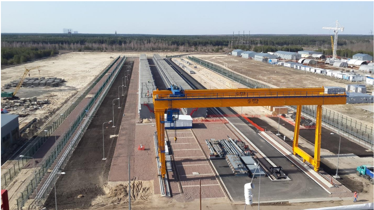
Aerial View Of The Construction Site
