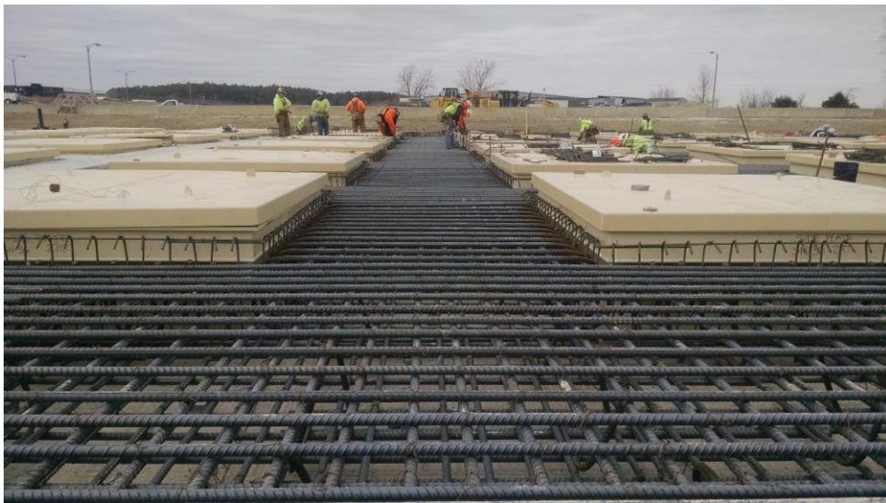
Rebar for the Top Pad (January 2015)
