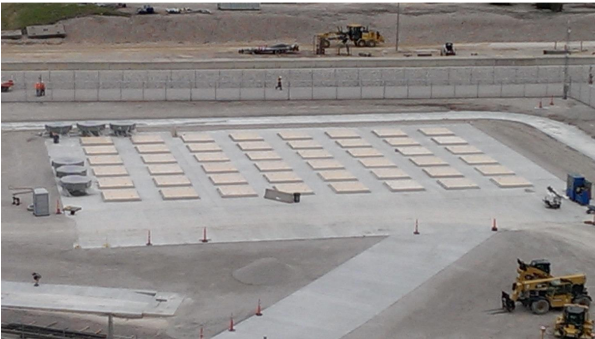
ISFSI Pad, Apron, and Heavy Haul Path completed (April 2015)
