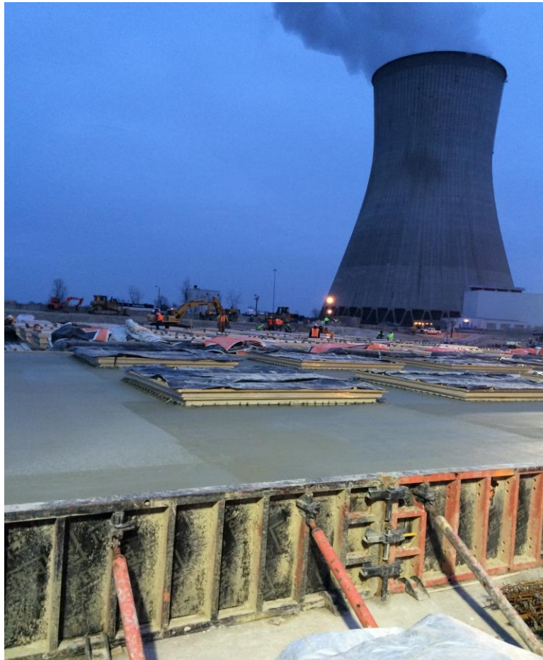
ISFSI Pad Concrete Pour Completed (January 2015)
