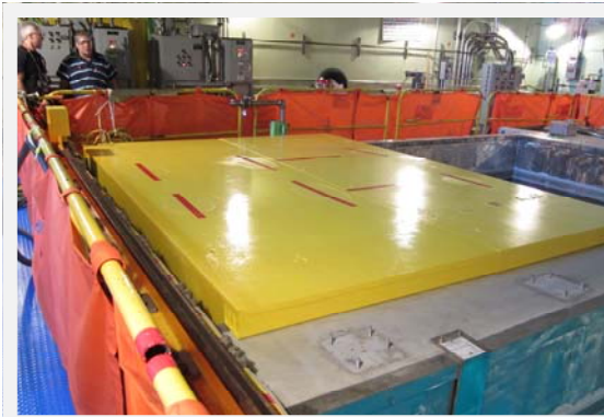
Load Drop Protective Cask Pit Platform
