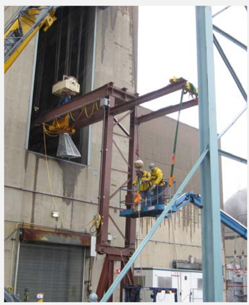
Installation of the Temporary Crane
