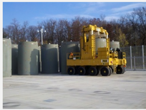
DC Cook ISFSI pad after completion of the site's first loading campaign
